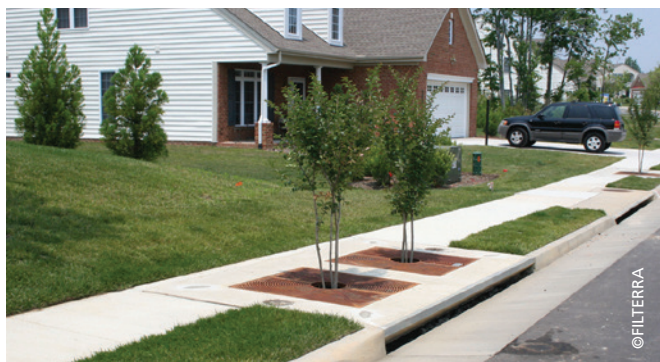
Linear stormwater tree pit
